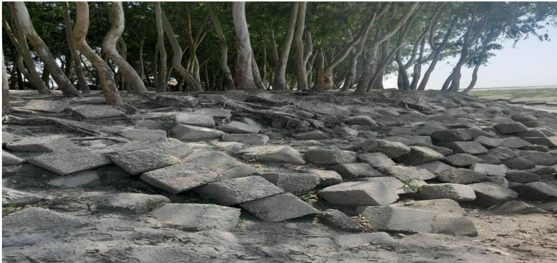
PictureFig.4. Concrete block ( Bojra ) adopted by GO
