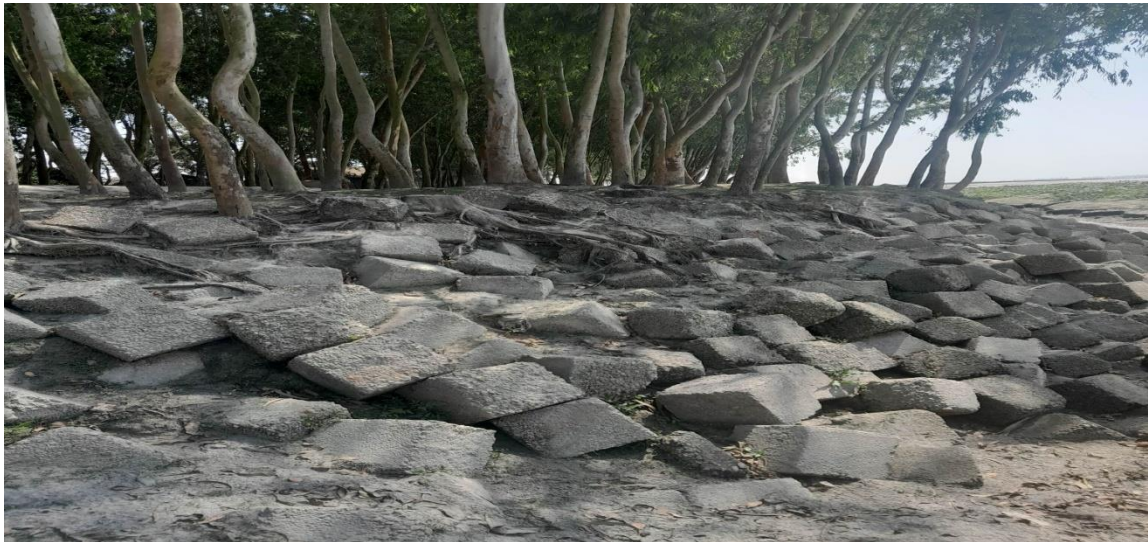
PictureFig.4. Concrete block ( Bojra ) adopted by GO
