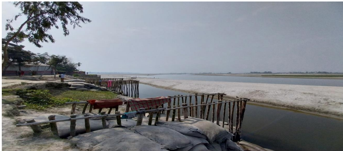
Picture Fig. 5. Bamboo fence piling/Bundal(Daldalia)
